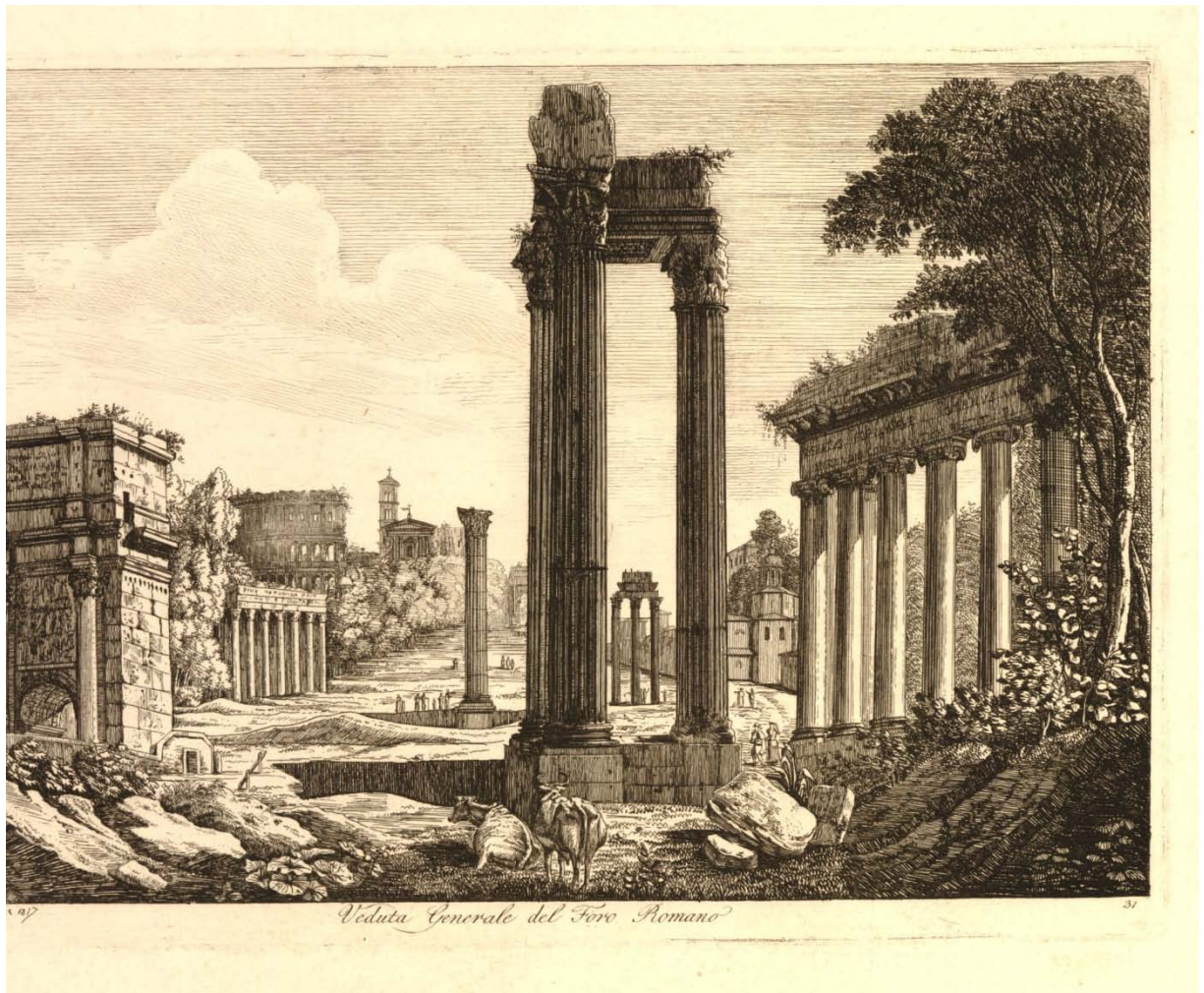
Fig. 3.2: The Column of Phocas can be seen in the middle ground of this veduta to the left of the three remaining columns of the Temple of Vespasian and Titus. This drawing was completed in 1817 and depicts the Duchess's ongoing excavation surrounding the Column of Phocas. Luigi Rossini, Veduta Generale del Foro Romano , 1817. British Museum, London.
